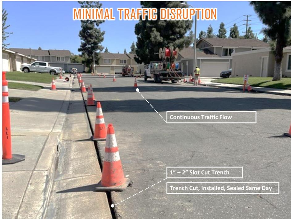
After the cement slurry has cured, SiFi would place a finish seal over the backfilled trench to match the color of the roadway surface. The installation process would have minimal impact to residential and commercial properties, as the trenching, conduit installation, and backfill takes place in a single day, with the finish seal installed shortly after.
